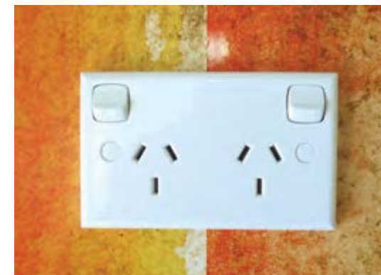
Power Point Installation – Front View
